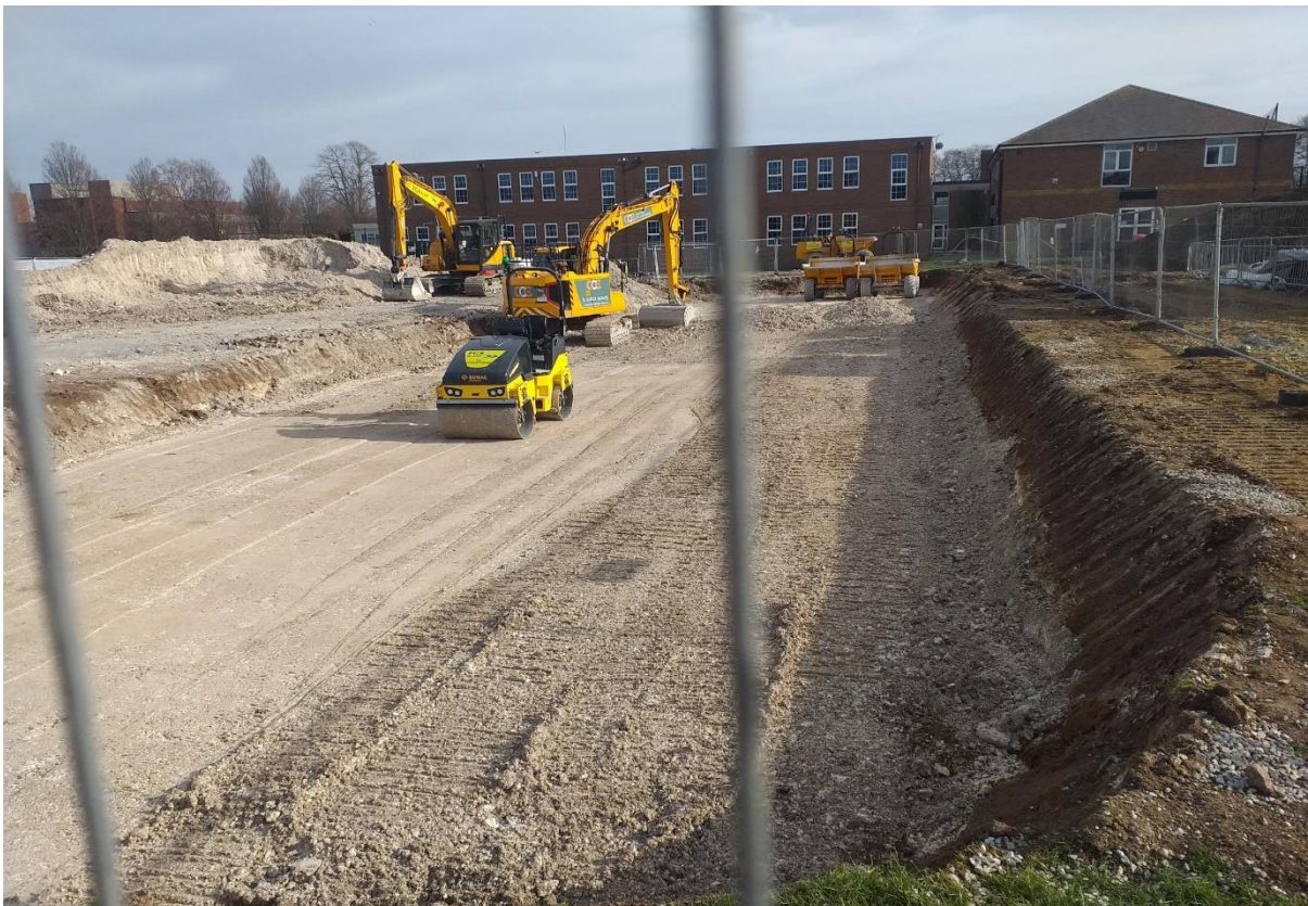
Attenuation tank being backfilled, rolled in layers of 250mm for strength
