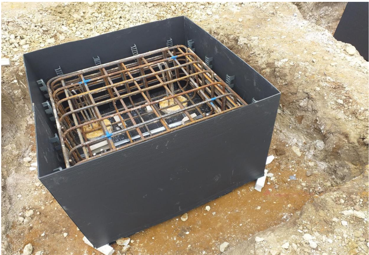
Reinforcement added to the top of the piles to form pile caps
