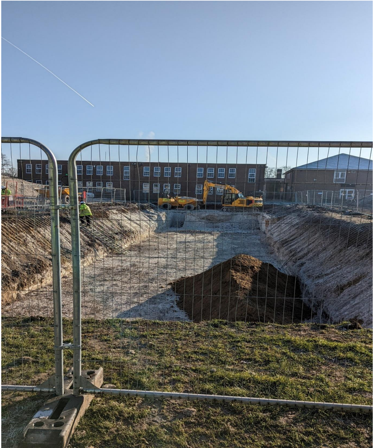
Attenuation tank dug to a depth of 3.5m
