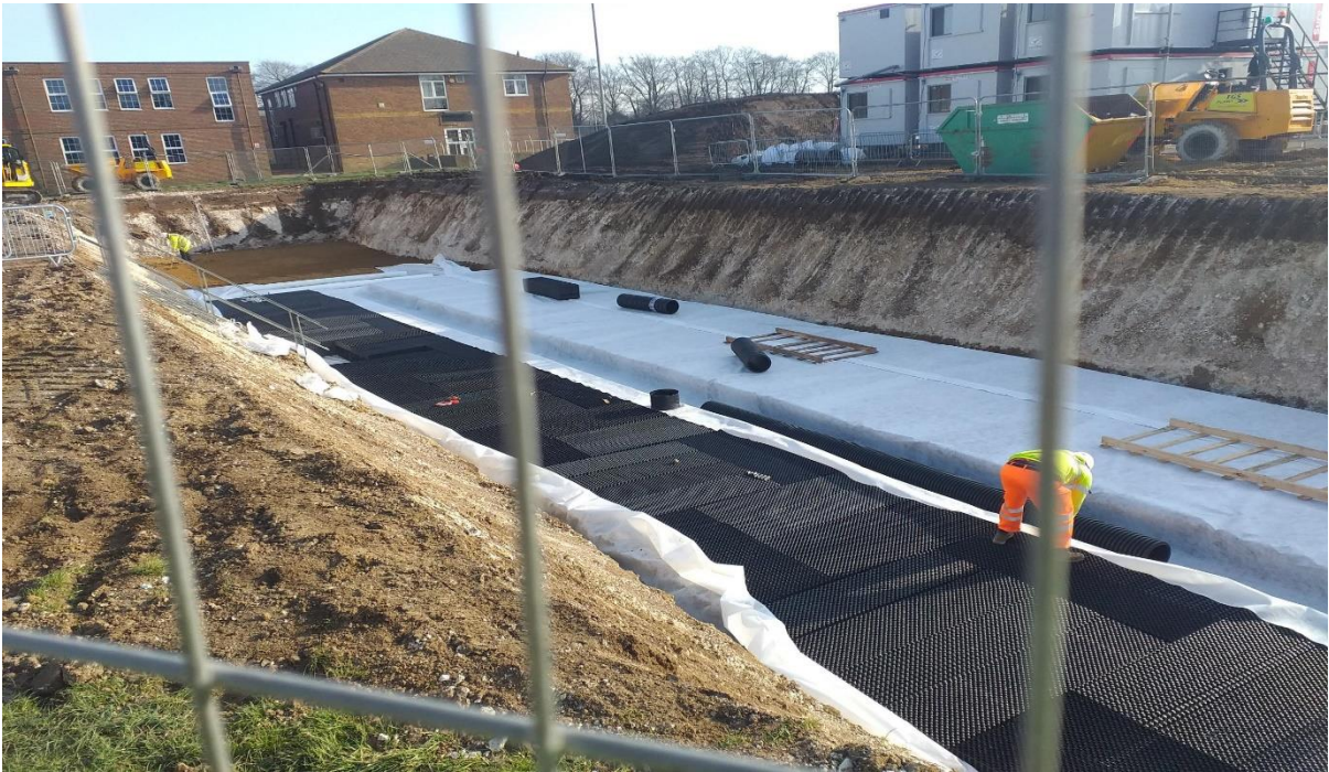
Attenuation tank being installed, to take all the rainwater away
