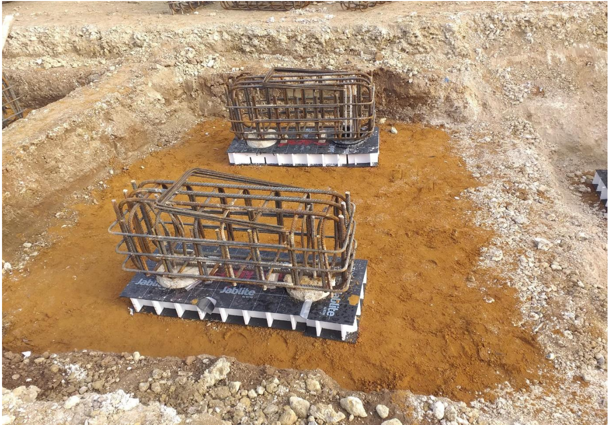
Reinforcement added to the top of the piles to form pile caps
