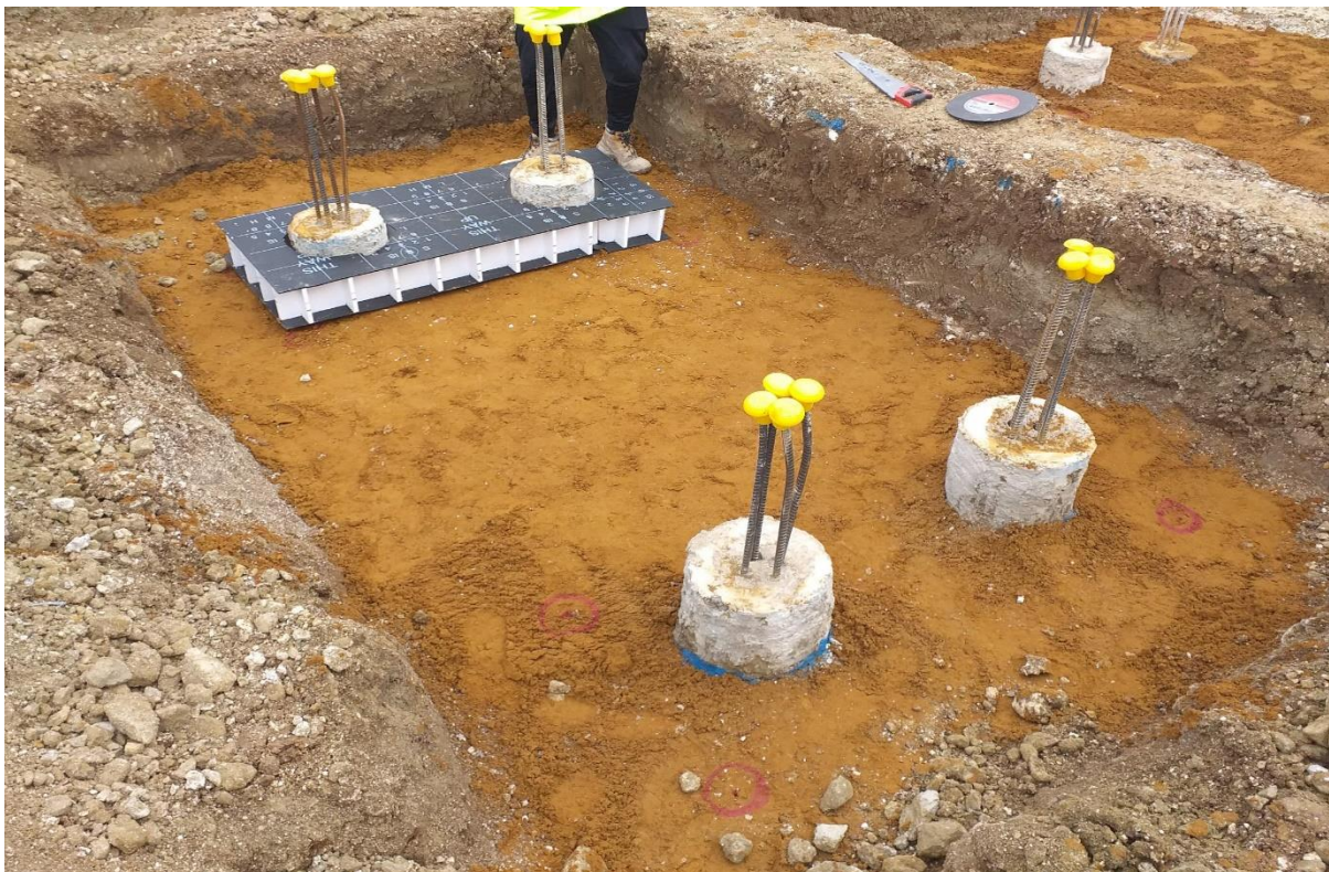
Here you can see the top of the piles with the reinforcement steel showing, a sand blinding and 100mm cellcore to allow for heave
