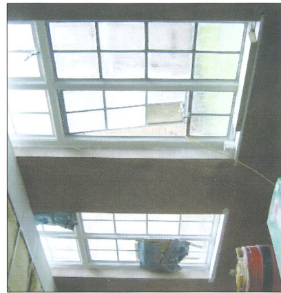
Room 1 looking towards the quadrangle
